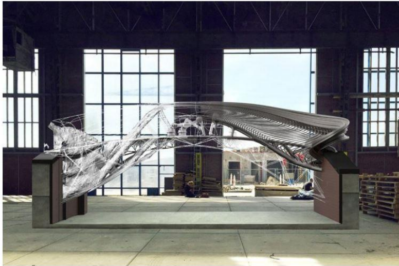
A rendering of the MX3D Bridge in the workshop. The bridge is being executed by robotic 3-D printers and will be completed in 2018. It will span an old canal in Amsterdam, connecting the technology of the future with the city's past. Joris Laarman Lab
